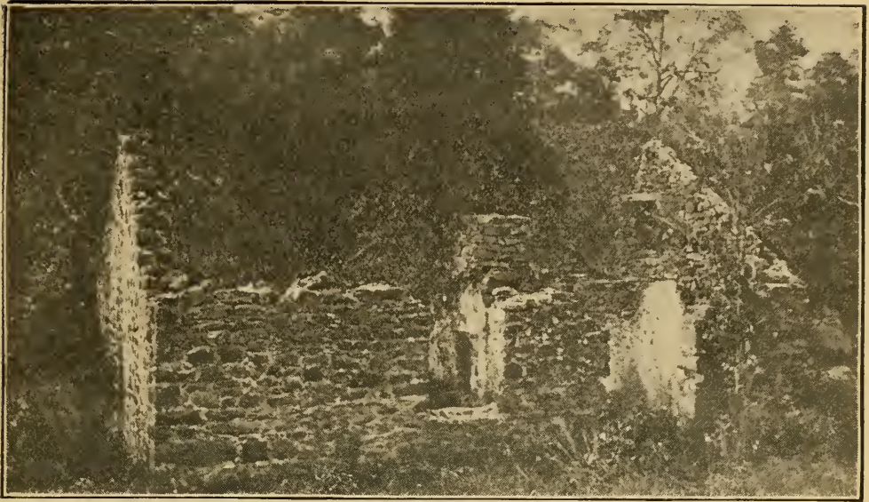
RUINS OF DRYHOUSE, USED BY MILLER BROS.
